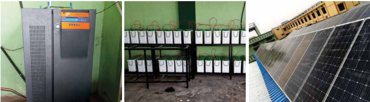
60KVA Off Grid System at Khurja, UP
